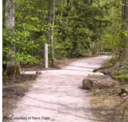
A natural tread consisting of a properly compacted limestone aggregate provides an excellent sustainable surface that can be easily repaired and maintained.
